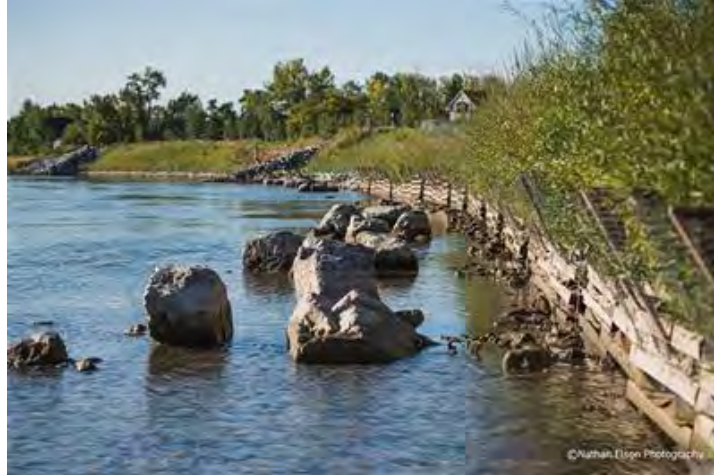
Figure 5: Bioengineering as an example of a natural measure that mitigates negative impacts of flooding and bank erosion.
