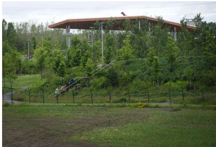
Figure 6: Example of park space integrated with flood barrier infrastructure.
